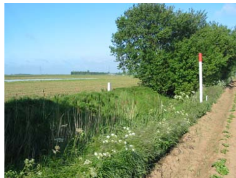
Typical Local Drain
