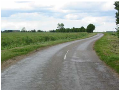
Typical Local Road
