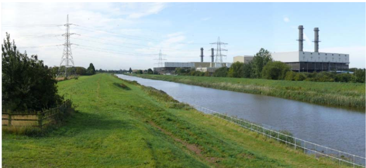
Photomontage of the proposed SEE (left) and the existing SECL Power Station (right) adjacent to the River Welland
